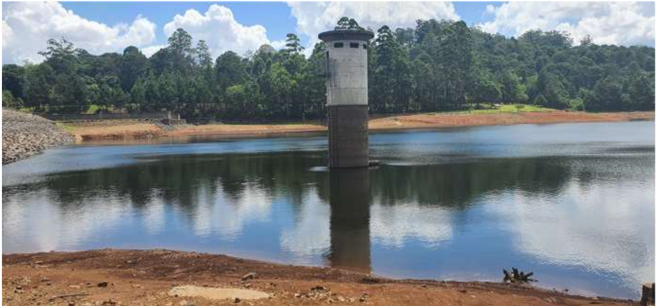
Figure 1: Status of Mulunguzi Dam on 18/12/2021. Source: SRWB-PRO
